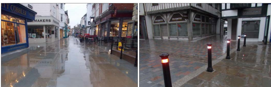
Substantial paving improvements were carried out at Fish Row, Salisbury
