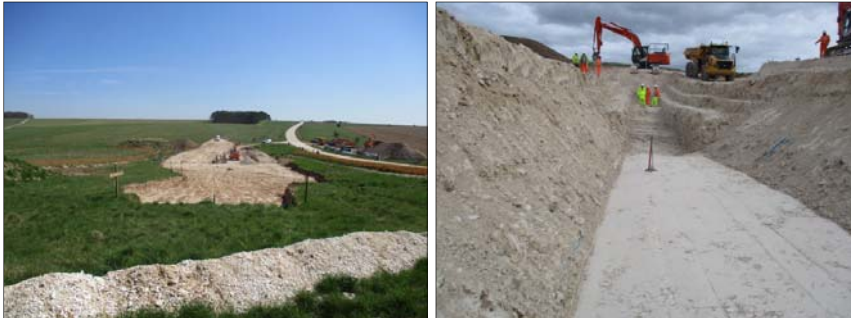
A substantial flood alleviation scheme is being constructed at Tilshead
