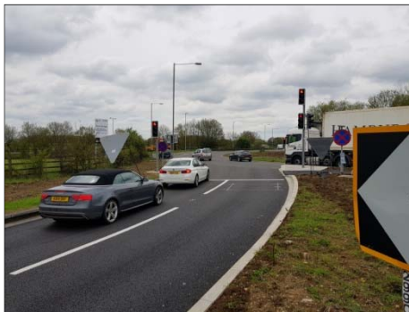
Improvements at the M4 junction 17 improved safety and reduced delays.
