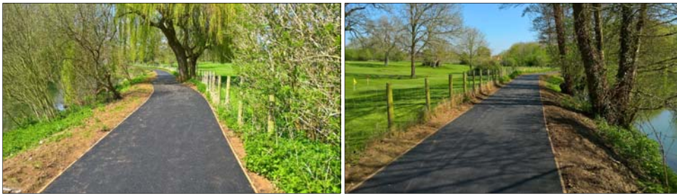
Cycle improvements undertaken at Monkton Park, Chippenham
